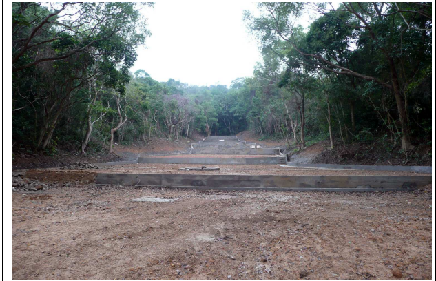
overview from entrance
