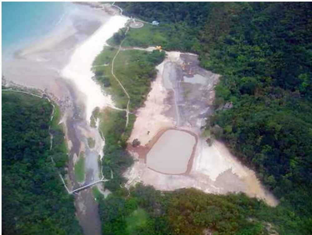
An aerial view shows a large-scale excavation behind the white-sand beach of Tai Long Wan.
